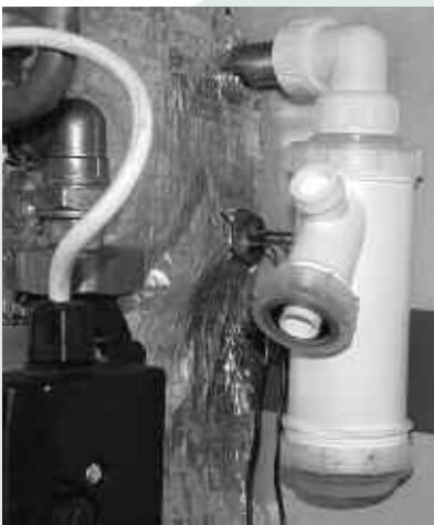
Figure 6-2: Condensate trap
