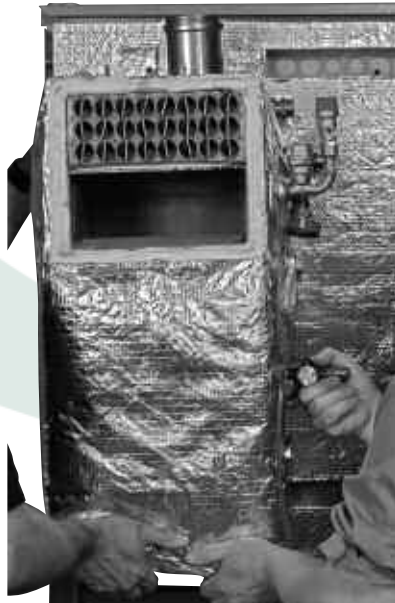
Figure 4-5: Lifting boiler out
