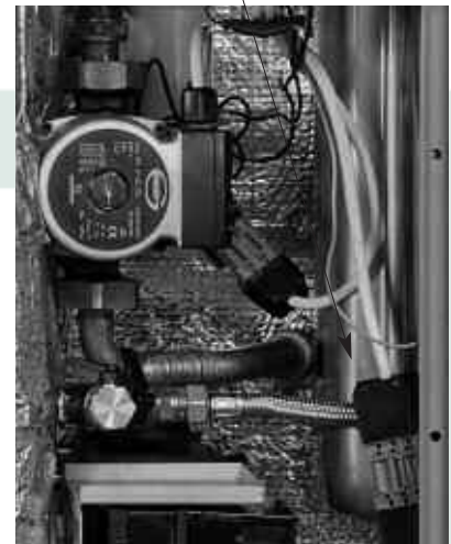
Figure 4-2: Removing thermostat phials
