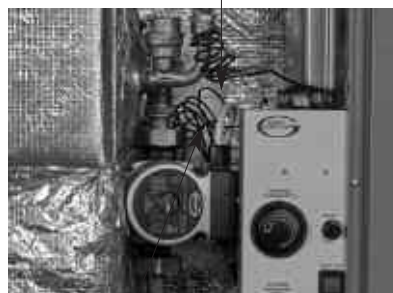
Figure 4-1: Condensate trap and thermostat phial location
