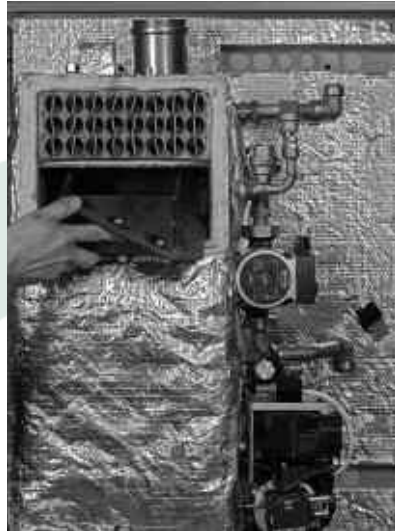
Figure 4-4: Baffle location
