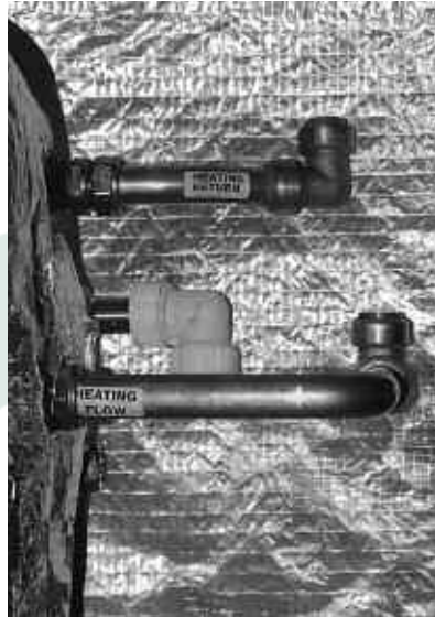
Figure 5-1: Non-system boiler flow and return connections
