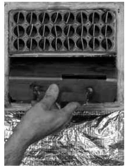
Figure 11-1: Removing the baffles
