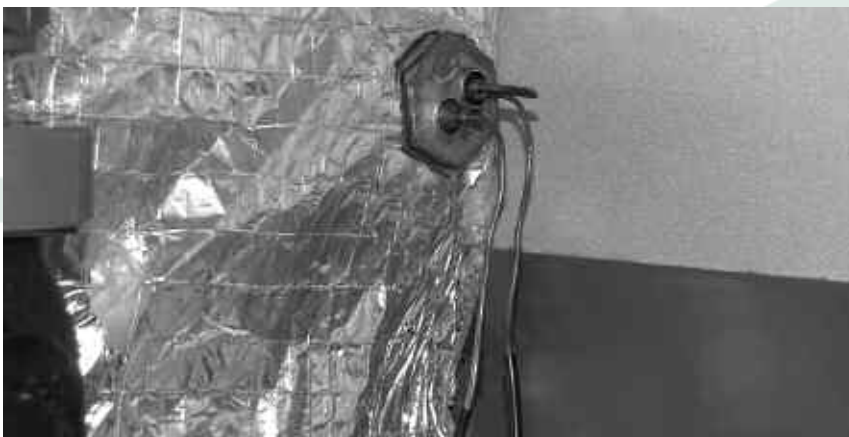
Figure 10-3: Thermostat phial position
